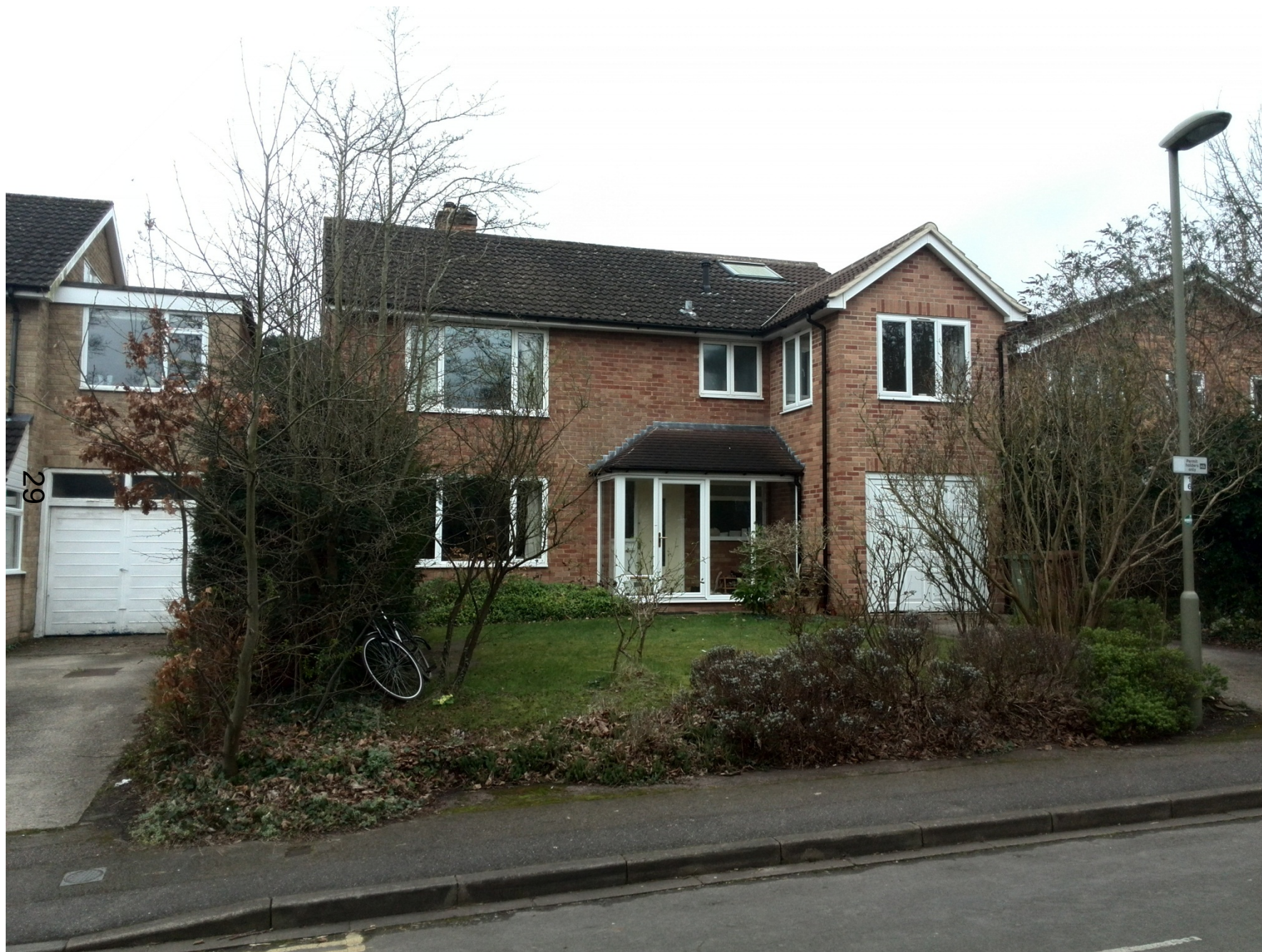
Front extension at 42 Franklin Road
